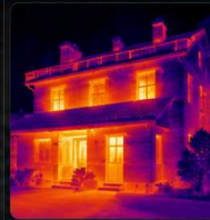
INFRARED THERMAL IMAGING
