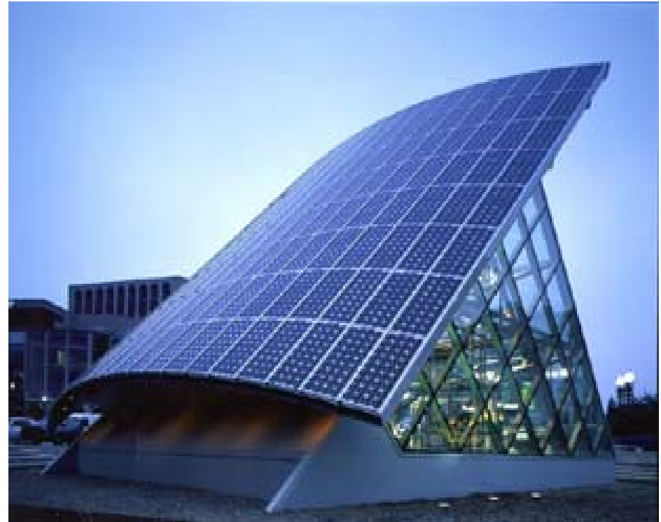
Buried contact solar cells used in building-integrated application at G8 Summit Building, England.
